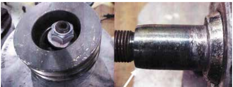
Examples of loose pulley damage on external fan type alternators
