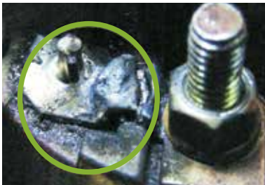
Good solder joint
